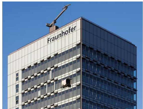
Fig. 70.6 SIRIUSc facade cleaning robot for automatic cleaning of high-rise buildings
