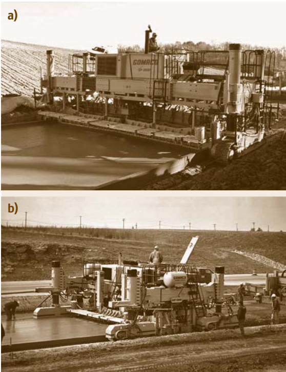
Fig. 61.1a,b Slip-form pavers: (a) screeding process, (b) idle workers during operation [61.26]
